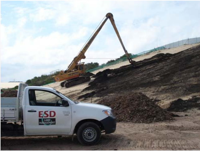
Steep and high sand dunes covered in growing media by ESD at Cronulla Business Park.
