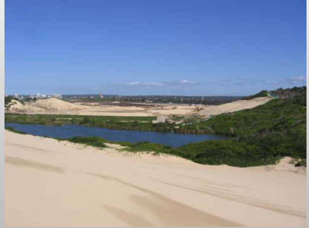
Cronulla Business Park—ESD works Stage 2.
