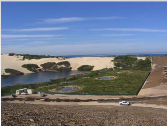
Construction work by ESD at Cronulla Business Park.
